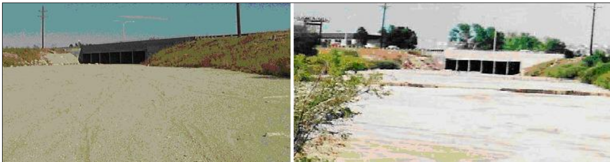
Exhibit 2-8. Sand Creek, Dry and Running, Downstream from Powers Boulevard
